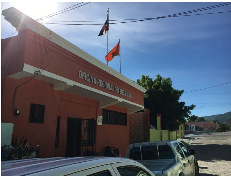
Figure 15. Regional Defensa Civil office in Barahona, Barahona Province, the Dominican Republic
